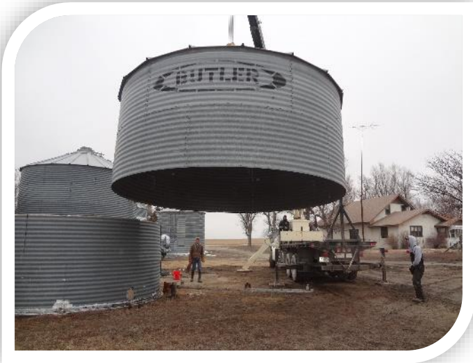
Grain bins being taken down in Palco, KS.
