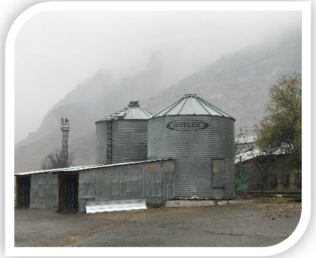
The same bins rebuilt in Kyrgyzstan!
