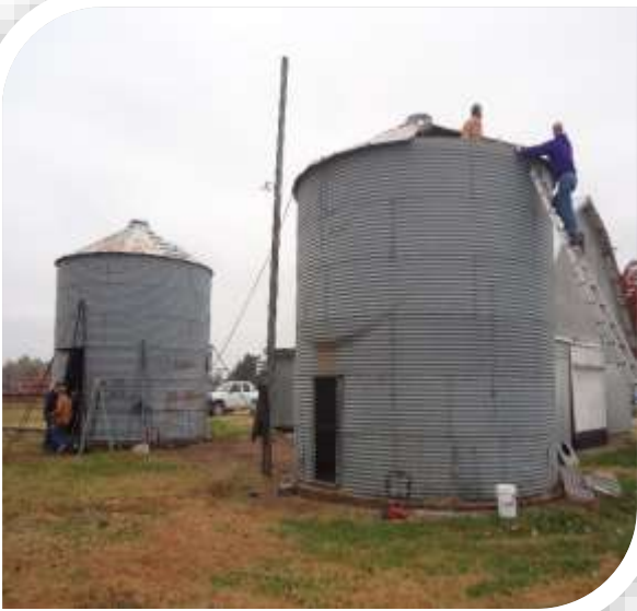
Grain bins being disassembled for shipment.
